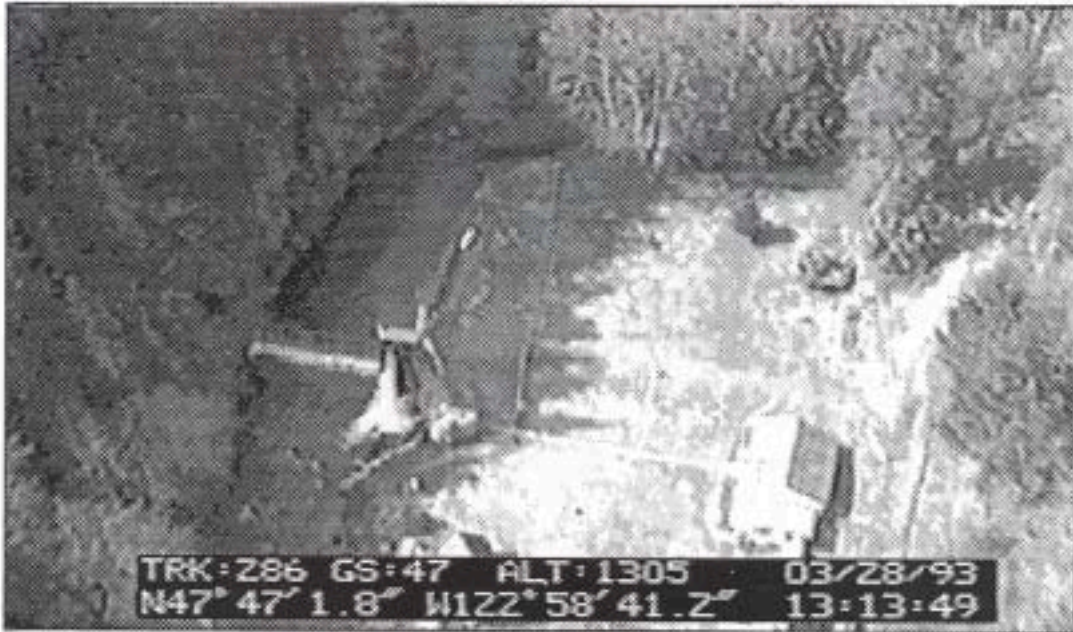
Figure 2.22 A view, looking west, of the diversion dam at RM 9.3, diverting water through a gravity pipeline for municipal and industrial use at Port Townsend.
